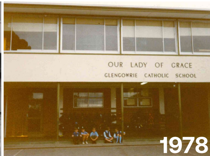
Three Room Addition This addition was to the original building, allowing for a new classroom, wet areas and withdrawal room.
